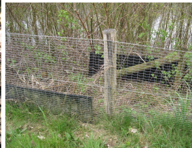
Figuur 5: Overlap amfibieënscherm is ca 30 cm.
