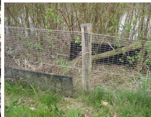
Figuur 5: Overlap amfibieënscherm is ca 30 cm.
